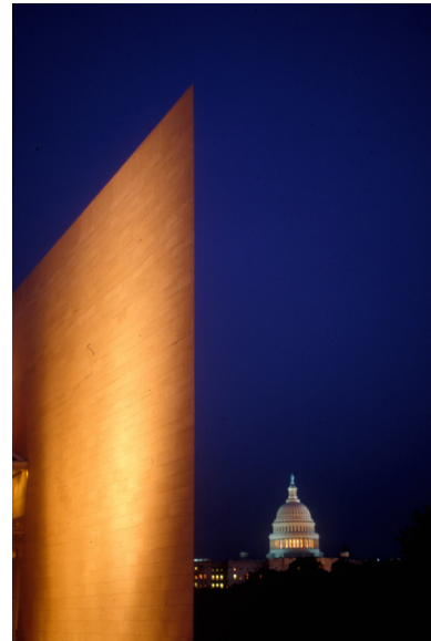
A view of the National Gallery of Art East Building and US Capitol dome at night. The “knife edge,” or signature southwest corner of the East Building, cleaves the air at 79.5 degrees to a height of 116 feet. It may be the sharpest corner of any building in the world. Photo © Dennis Brack/Black Star. National Gallery of Art, Washington, Gallery Archives
