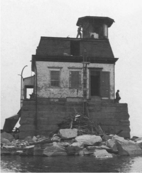
fig. 18. Workmen dismantling the Colchester Reef Lighthouse, c. 1870, in preparation for its move ashore, 1952 [Shelburne Museum]
