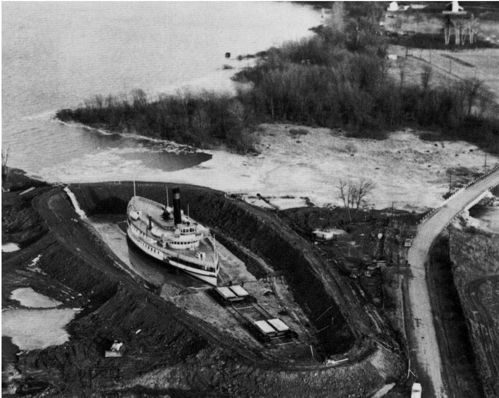
fig. 20. A 450-foot-long basin is flooded in order to position the Ticonderoga over the specially constructed railroad carriages that will transport it across several miles of frozen marsh to the museum grounds [Shelburne Museum]
