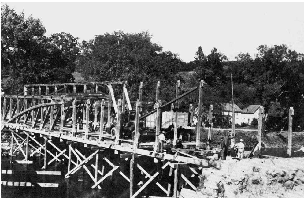
fig. 23. The covered bridge from Cambridge is reassembled over a specially built pond on the Shelburne Museum grounds, 1950 [Shelburne Museum]
