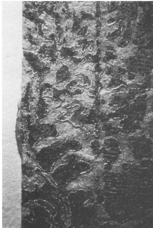
27. Detail, fig. 5, showing the deteriorated and blanched resin layer
