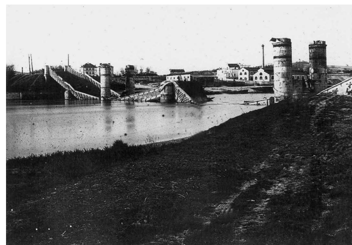
Fig. 27. Photograph of the railroad bridge at Argenteuil, damaged during the Franco-Prussian War, c. 1871
