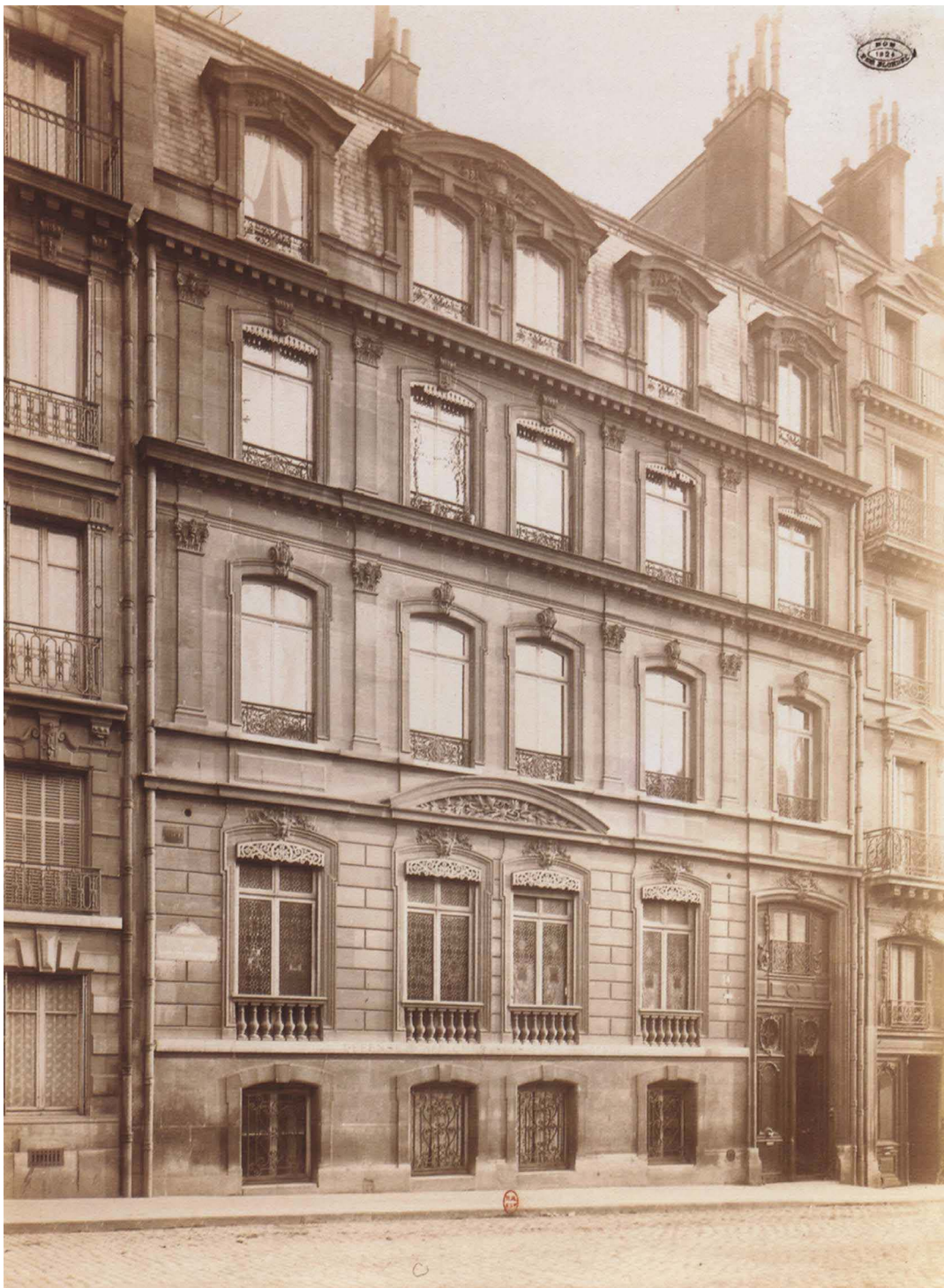
42 Façade of 4 rue de Saint-Petersbourg, albumen print, c. 1870, Bibliothèque nationale de France, Estampes, Paris (cat. 68); the house was built in 1864 and Manet's studio lay behind the four leaded windows with stone balustrades.
