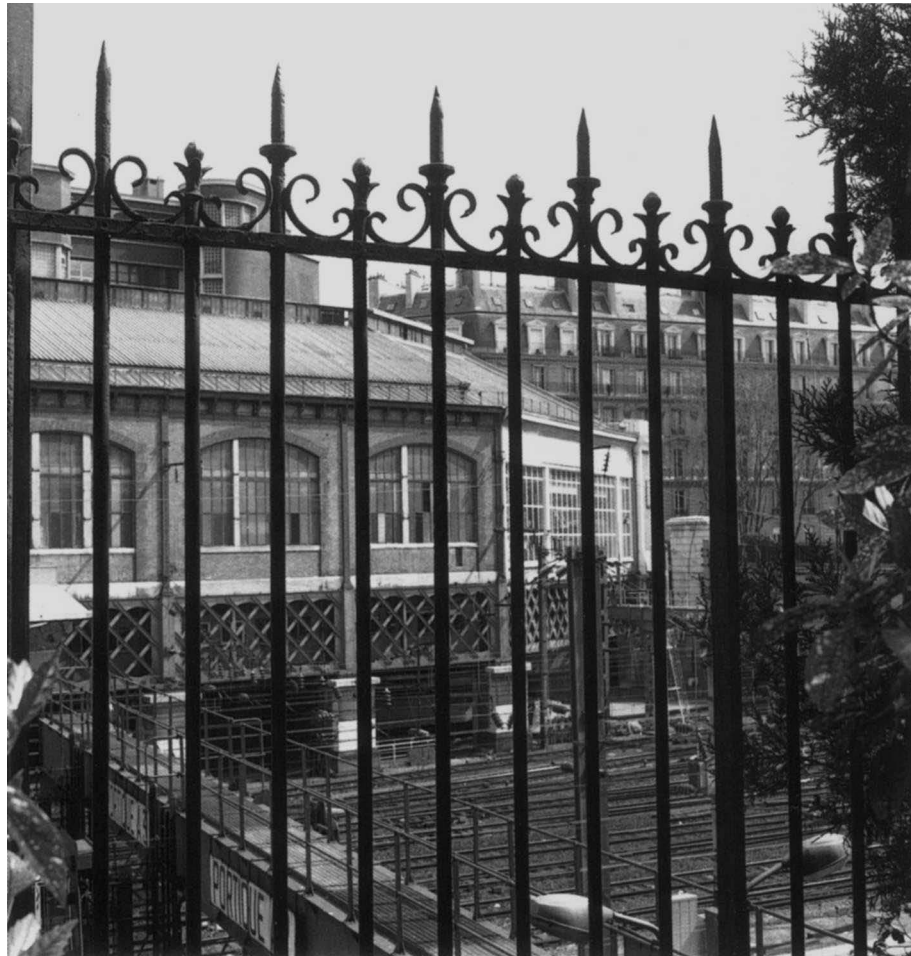
54 View from the rue de Rome garden, photo, Musée d'Orsay, Paris; the 1886 parcels depot and 1936 postal building blocking the view of 2 and 4 rue de Saint-Pétersbourg.
